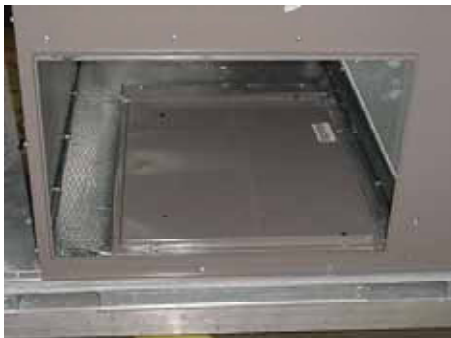
Figure 20: Discharge Panel In Place
